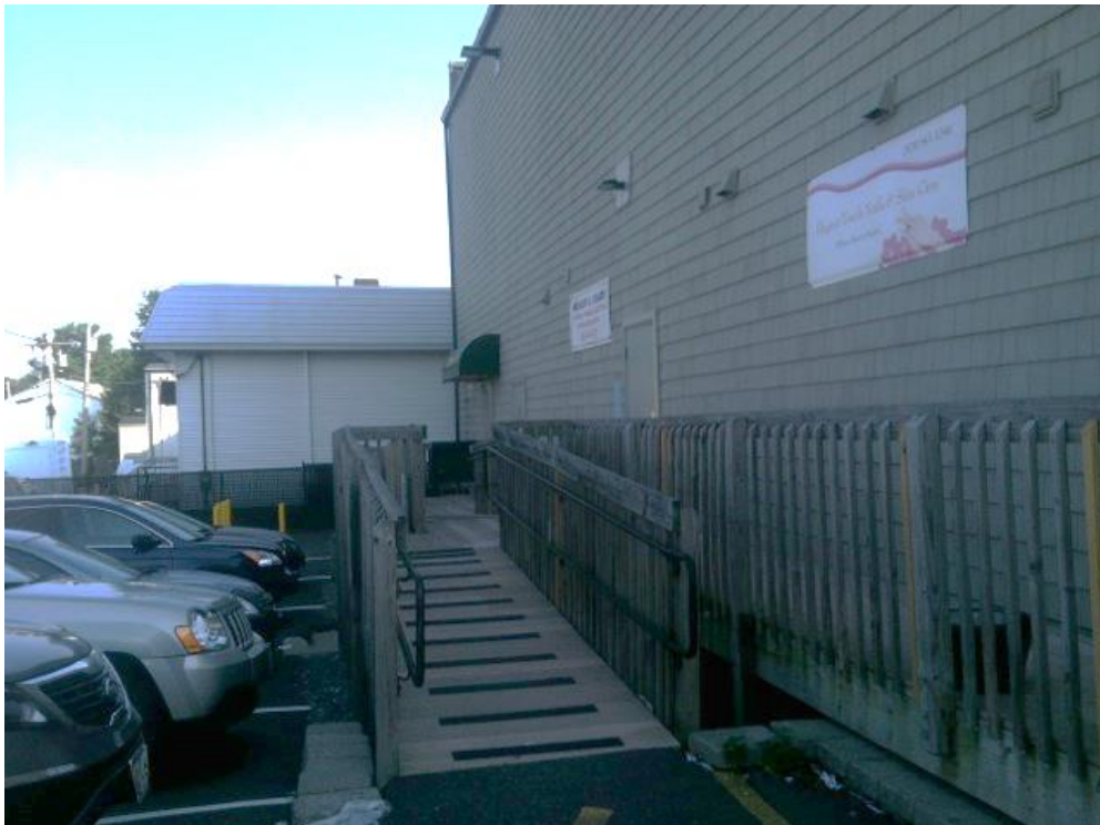
FIGURE 1 New Ramp behind the Boch Building
