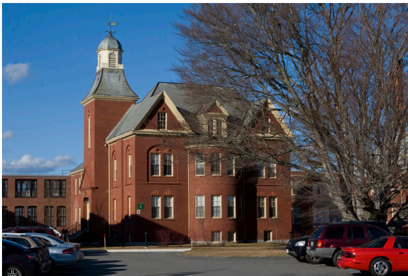
Figure 5-18 and 5-19. The Foxborough State Hospital campus is listed on the National Register, as part of a thematic, multiple properties nomination.
