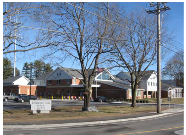
Figure 4-9. The Public Safety Building at Chestnut Green. Source: http://foxboroughpolice.com/
