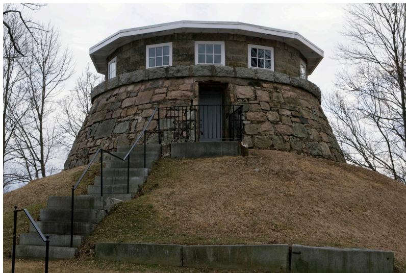
Figure 5-29. The Union Straw Works Reservoir on the site of the former Powder House.
