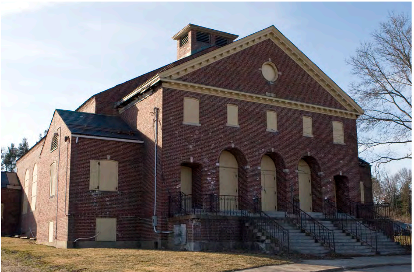
Figure 4-15. The Auditorium Building on Payson Road is currently vacant.
