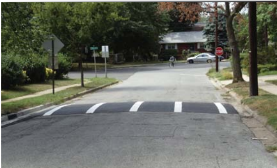
Figure 2-7. Speed bumps can be used to slow traffic, making residential streets safer.
