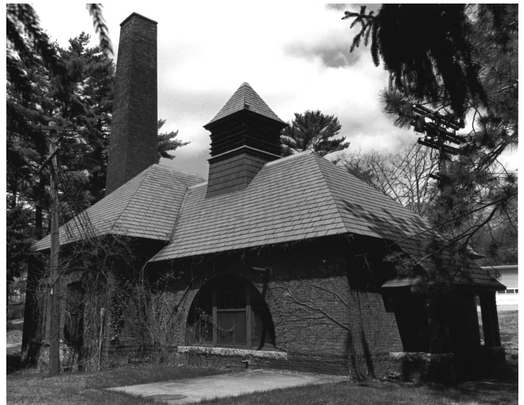
Figure 5-27. Foxborough Pumping Station, 2003.
