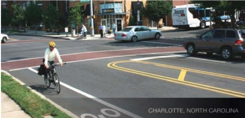
Figure 2-8. Complete Streets. A 'complete street' in Charlotte, NC with plantings, crosswalks, and bike lanes for improved pedestrian and bicycle use.
