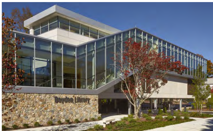
Figure 4-8. New addition at Boyden Library, Foxborough. Source: http://llbarch.com/projects/featured/boyden-library/
