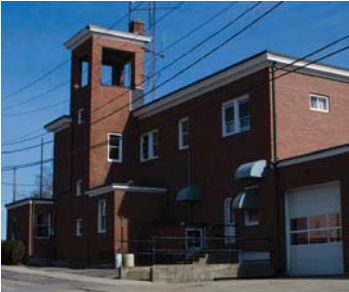
Figure 4-3: The fire station site is a potential redevelopment site for an education, youth or cultural use.
