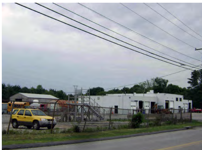
Figure 4-10. The Foxborough Public Works Building.
