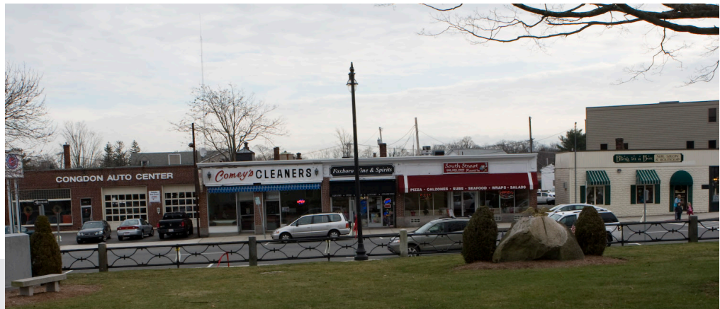
Figure 5-13 to 5-16: South Street and Central Street in Downtown Foxborough today.
