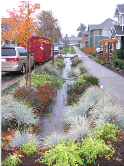
Figures 4-3 & 4-4: Bioswales to remove silt and pollution from stormwater runoff integrated as a landscape feature on a residential street.
