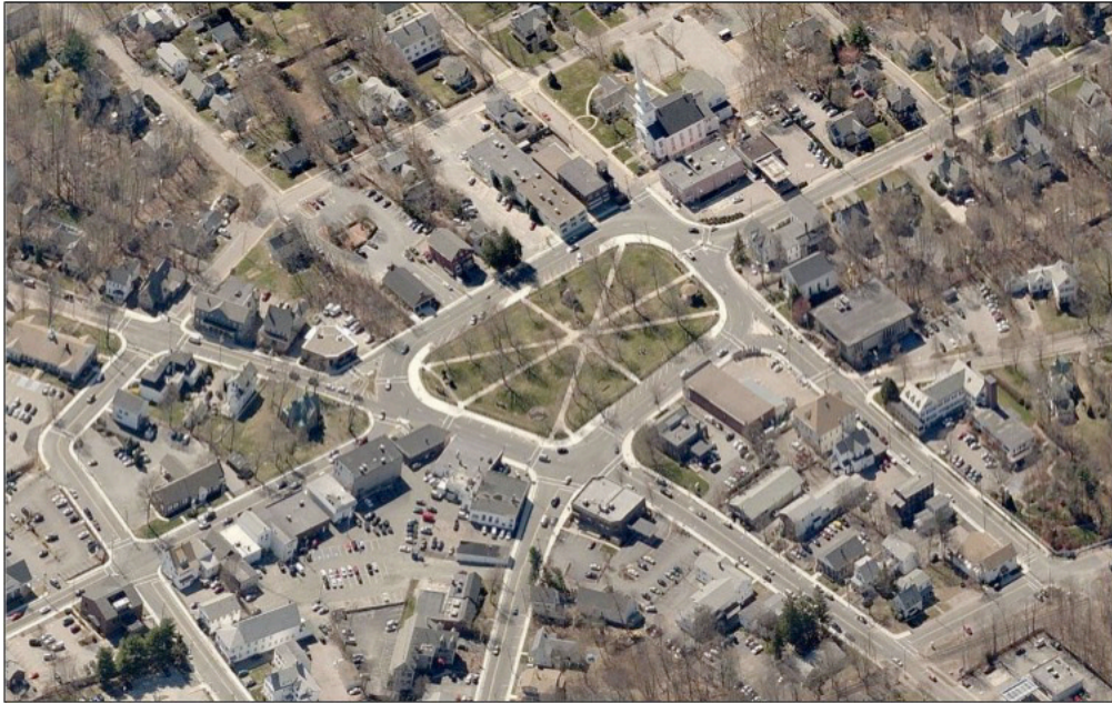
Figure 6-4: Aerial view of Downtown Foxborough
