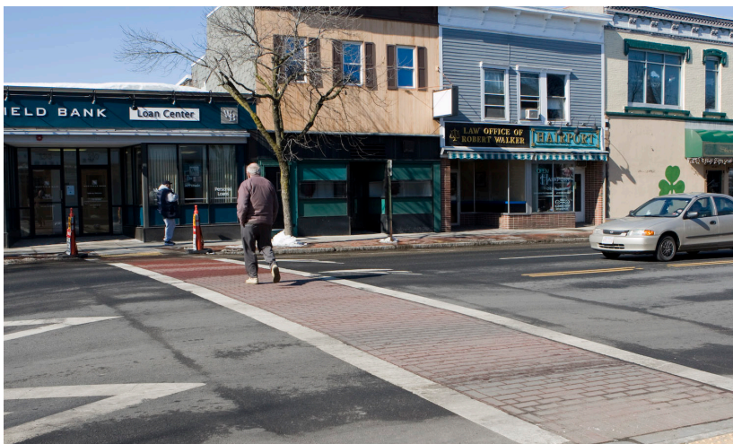
Figure 6-13: Raised, mid-block crosswalk provides a visible, safe crossing for pedestrians in Downtown, while slowing traffic. Pictured at the left is a raised crosswalk on Route 202 in Downtown Westfield.
