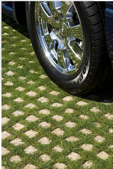
Figure 6-8: Grass paver system provides a permeable surface.
