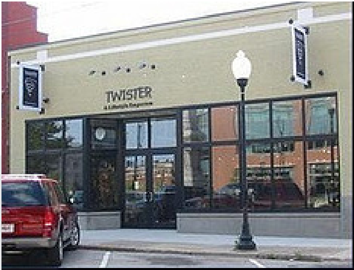
Figure 7-16: A simple storefront with a clean, modern look that respects traditional storefront elements.
