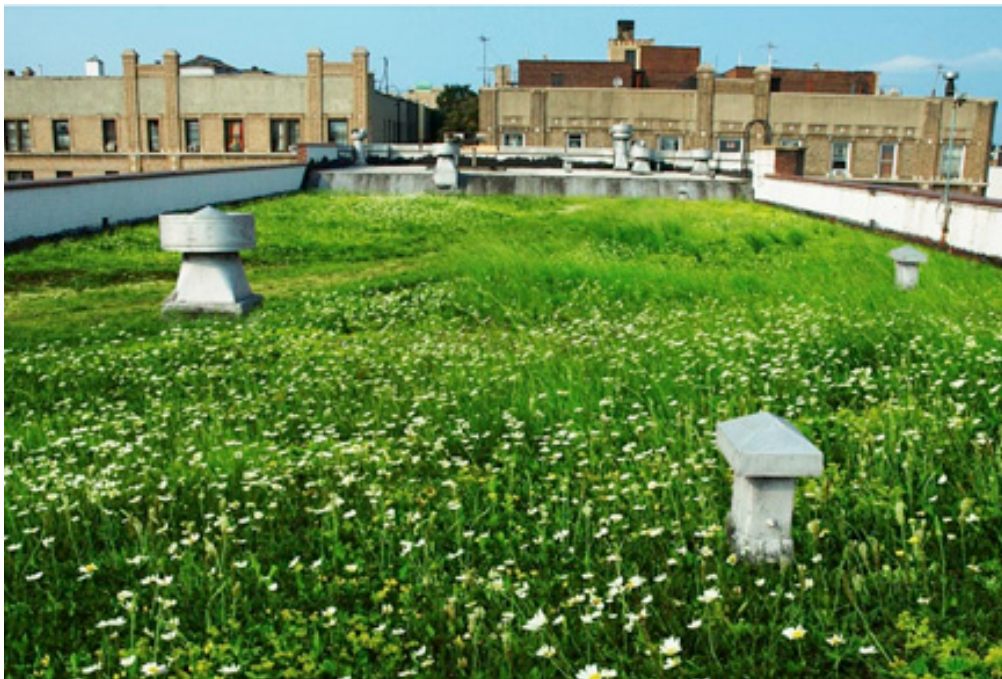
Figure 4-5: A ‘green roof’ on a downtown building helps lower air temperatures in the immediate area and reduces heat island effect. In addition it helps absorb rain water and provides added insulation for the building.
