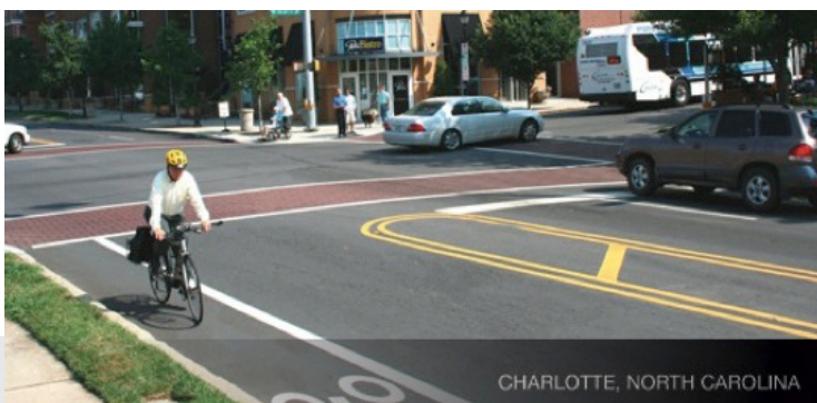
Figure 6-10: A ‘complete street’ in Charlotte, NC with plantings, crosswalks, and bike lanes for improved pedestrian and bicycle use.
