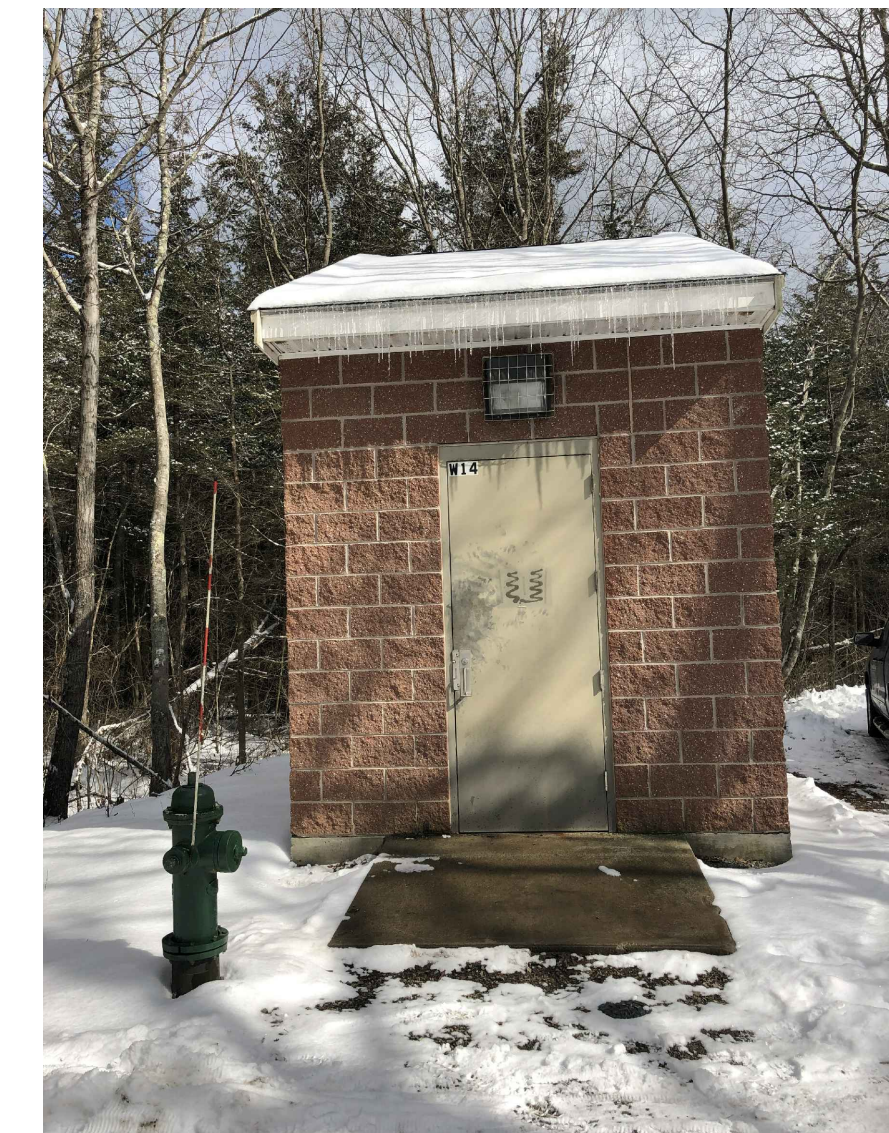
PHOTO 2 SCALE: N.T.S. WELL STATION 14 LOOKING EAST
