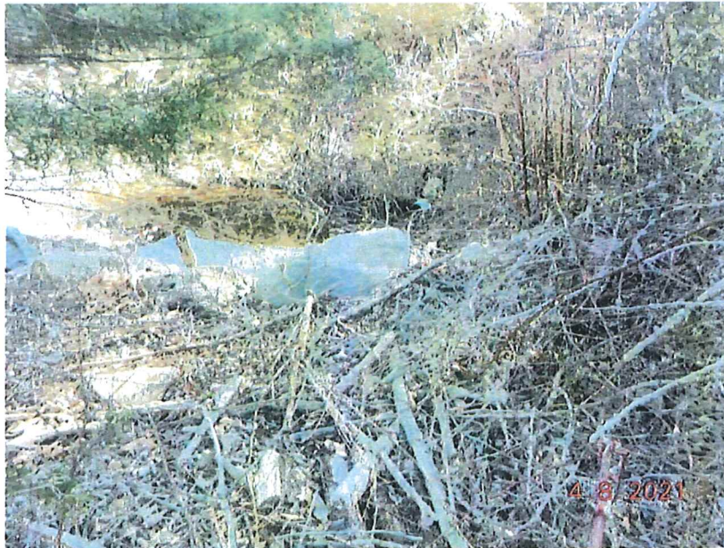
Photo 2 – Excavated Area on 217 Cocasset St. showing PVC pipe emanating from 227 Cocasset Street. Looking northwest from 217 Cocasset Street.
