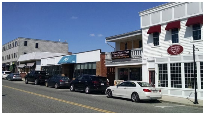
On-Street parking along central street is typically occupied while spaces in the lot behind the businesses remain open. With the installation of wayfinding signage in 2021 the lot has experienced and increase in use
