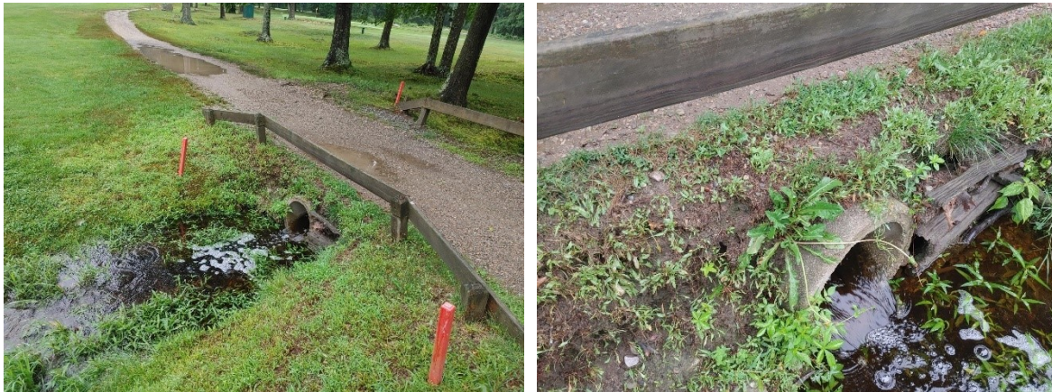
Both Photographs: Views of existing culvert and wooden headwall. July 2, 2021.
